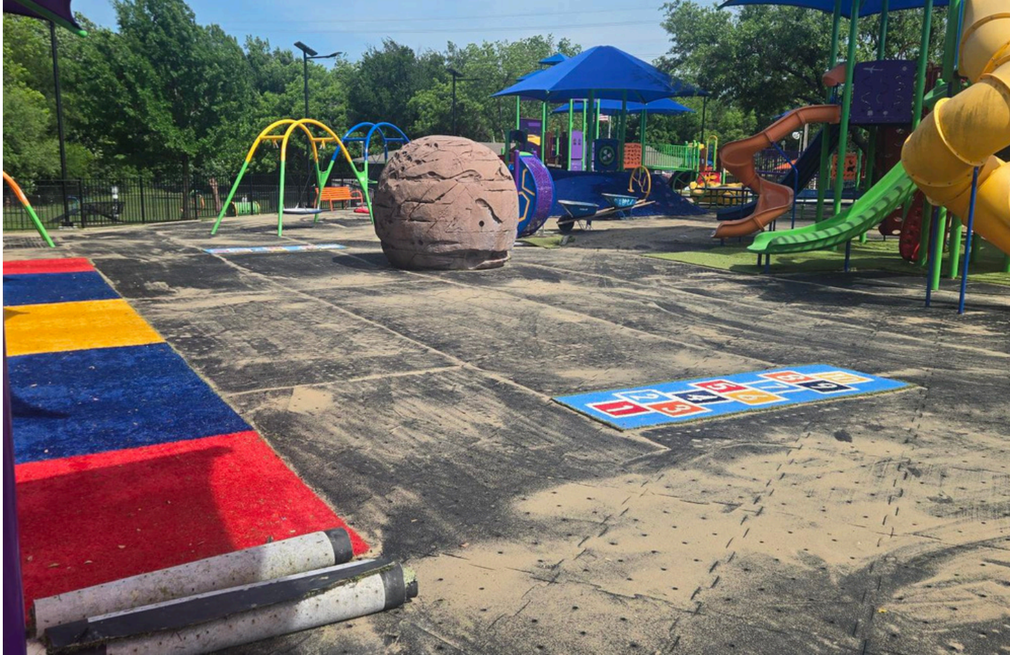
KIDZONE ARTIFICIAL TURF REPLACEMENT
